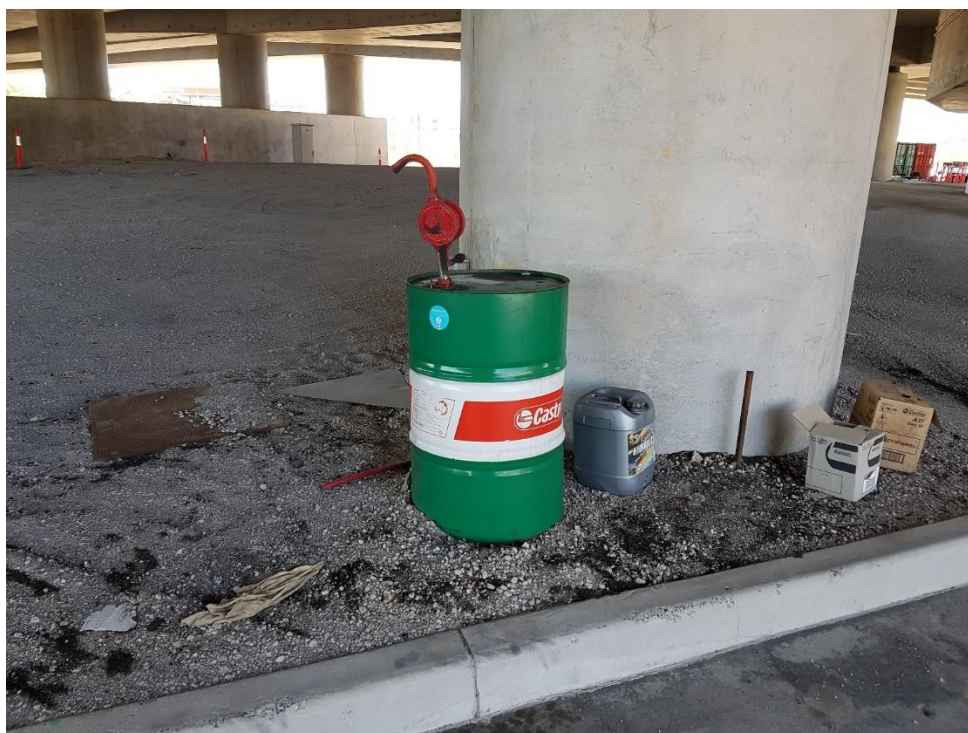
Plate 5A: Unbundled fuel drum below Ramp D (Before Photo)
