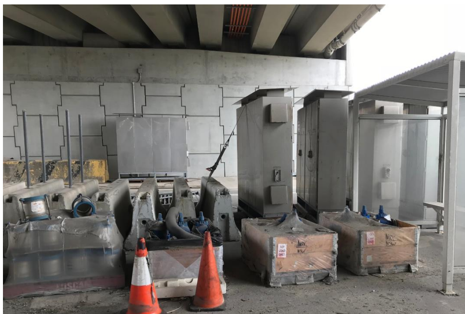
Plate 10B: Unbunded waste oil IBC removed from under Ramp D for disposal (After Photo)
