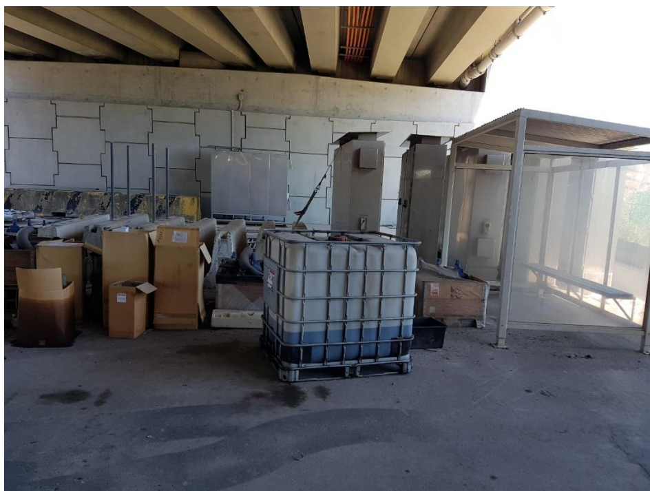
Plate 9A: Unbunded waste oil IBC under Ramp D (Before Photo)
