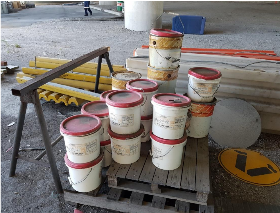
Plate 7A: Unbanded chemical containers under Ramp D (Before Photo)
