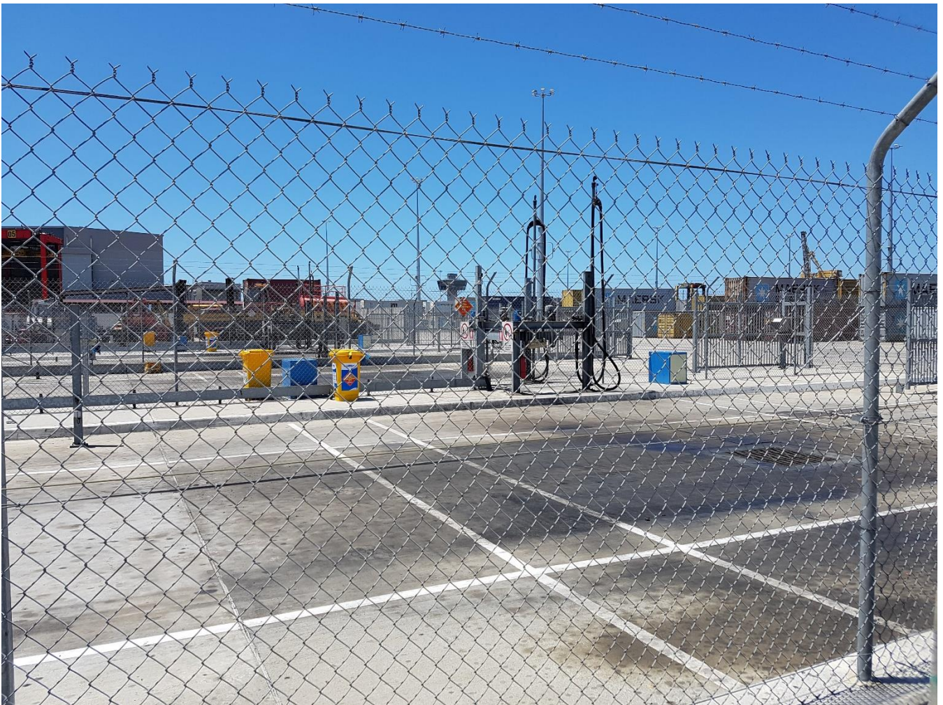
Plate 19: Internally draining Straddle Carrier refuelling bay with spill kits present
