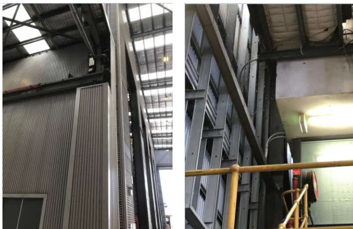
Photo 6.13.1: Use netting to limit access into the Maintenance Workshop.
