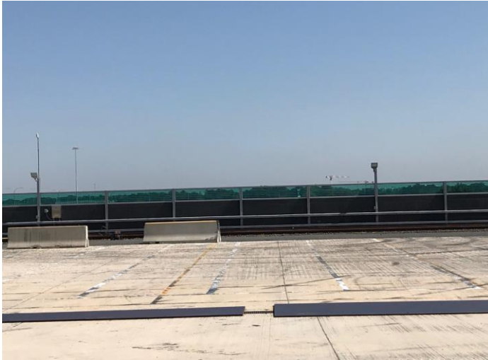
Photo 6.10.1: Noise attenuation wall positioned on the Northern side of the Patrick terminal, between Hutchison’s rail siding and the Penrhyn Estuary
