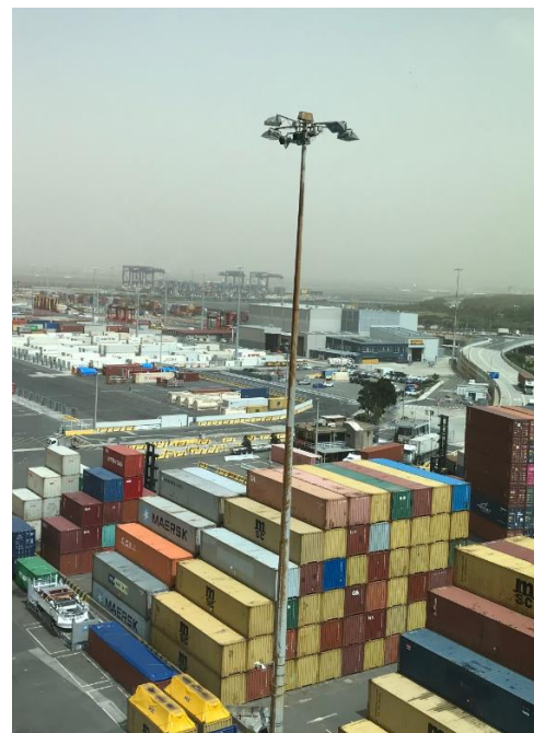
Photo 6.13.2: Visual inspection of light poles for nests
