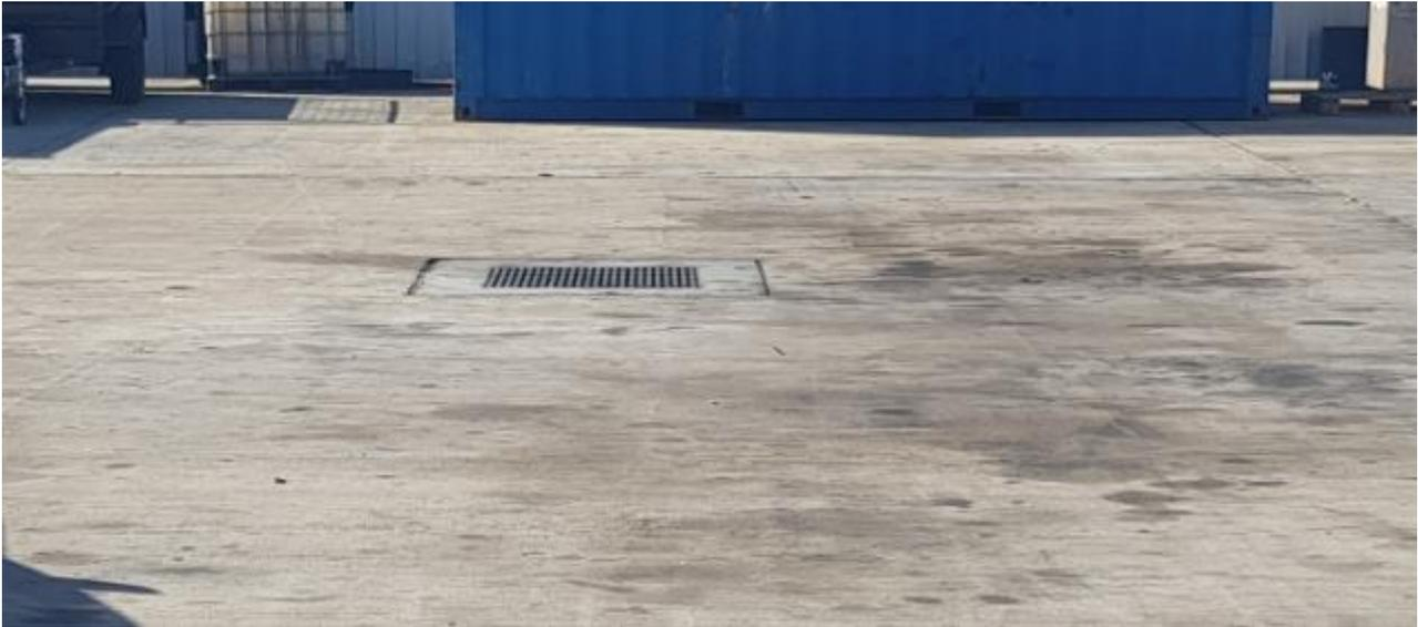
*Site Photo 5 Example of unmarked stormwater pit.*
