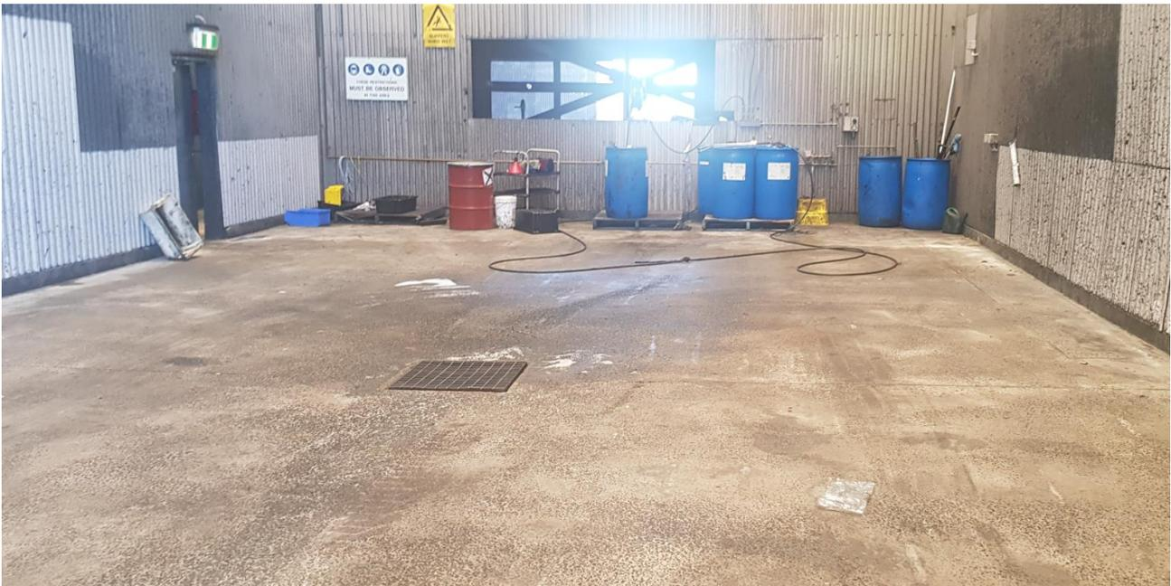
*Site Photo 3 Wash bay that drains to pit connected to wastewater treatment plant.*
