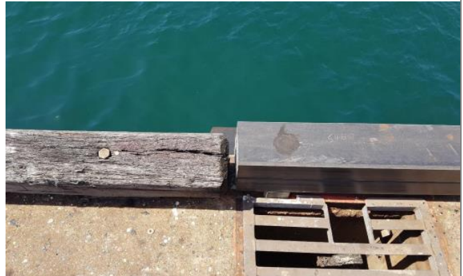
Photo 6.8.2: Wooden stringers (left) being replaced with recycled plastic stringers (right)
