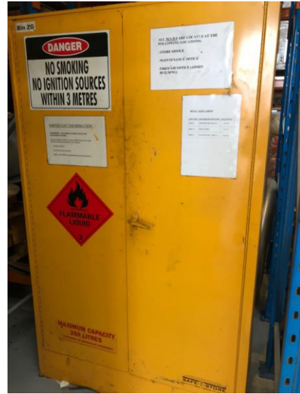
Photo 6.9.2: Flammable liquids cabinet
