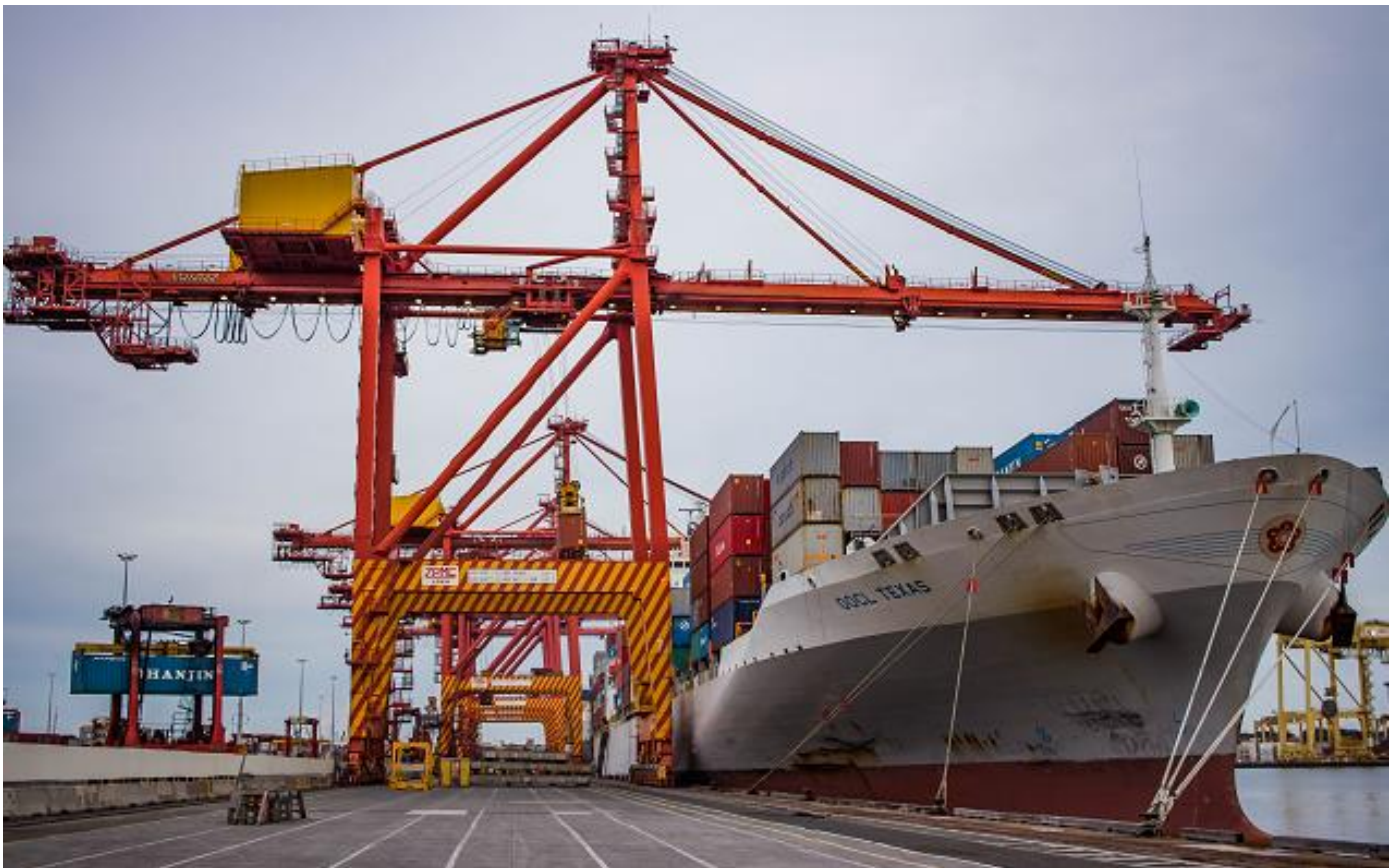
Courtesy of Bob Wood – OOCL Texas berthed at Patrick's Port Botany Terminal, 2017
