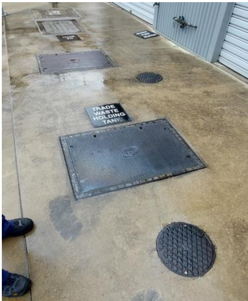
Site Photo 7 Liquid waste holding pit (Maintenance).
