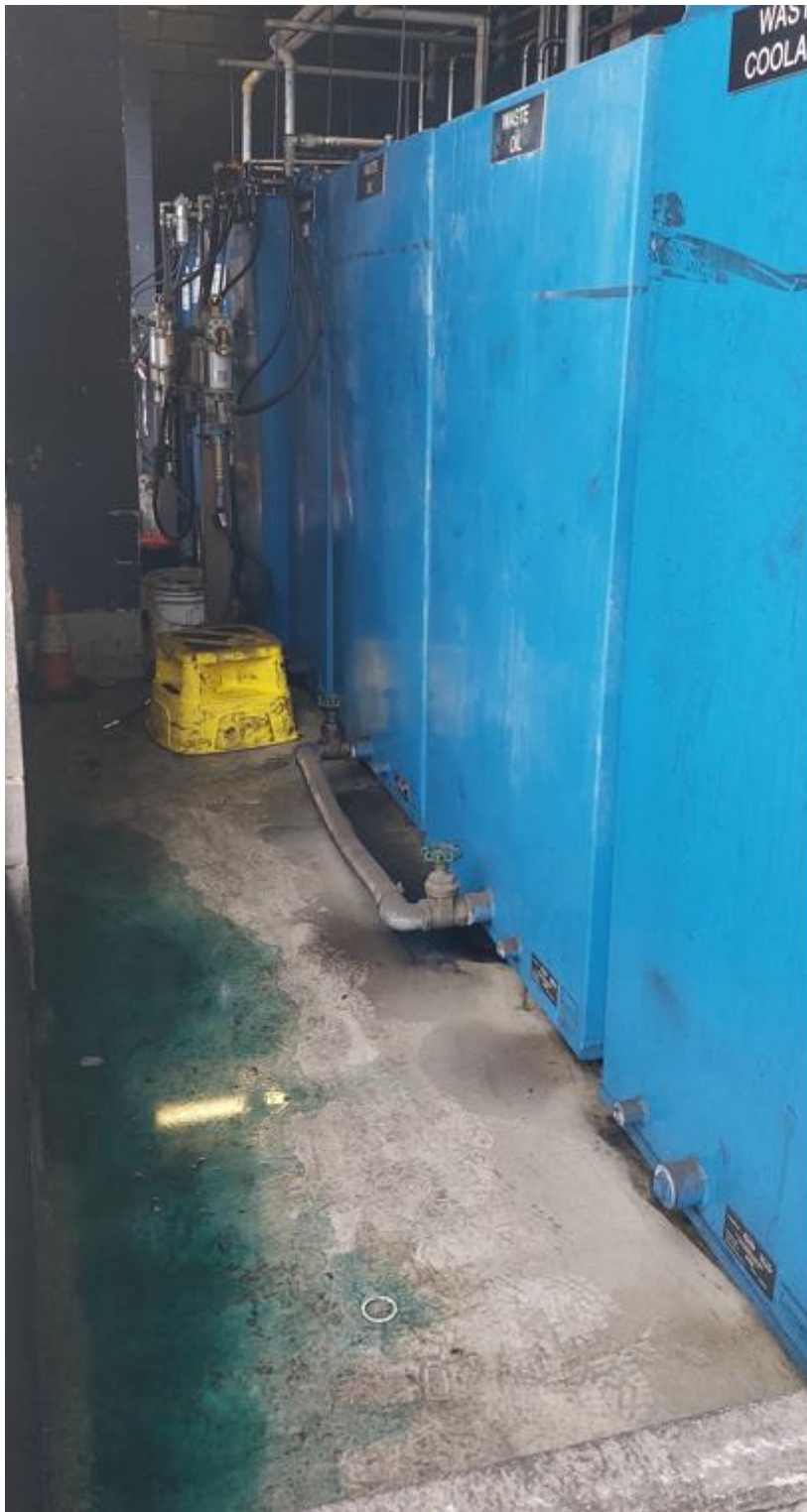
Site Photo 1 Waste oil and coolant storage point (Maintenance).
