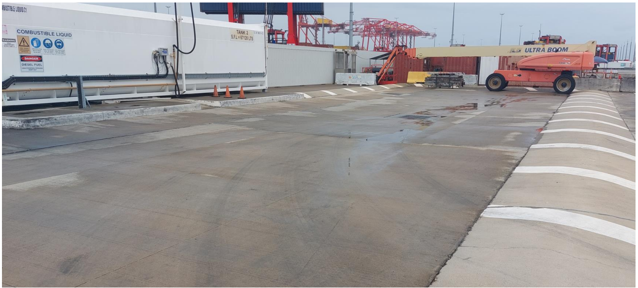
Site photo 11 Mobile plant refuelling bay
