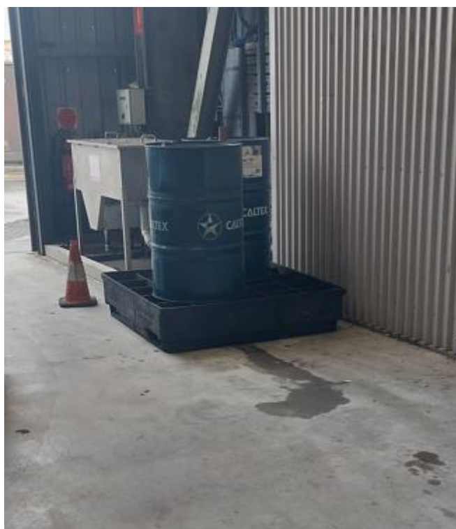
Site Photo 3 Drums in the Maintenance workshop stored on pallet bund whilst in use.
