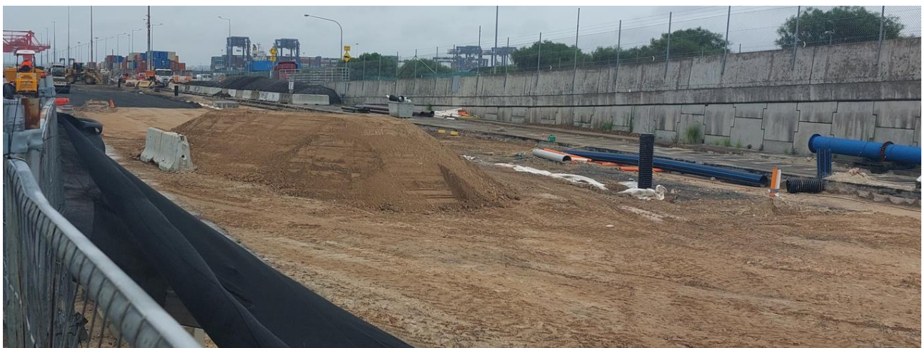
Site Photo 8 Rail construction area (under separate approval).
