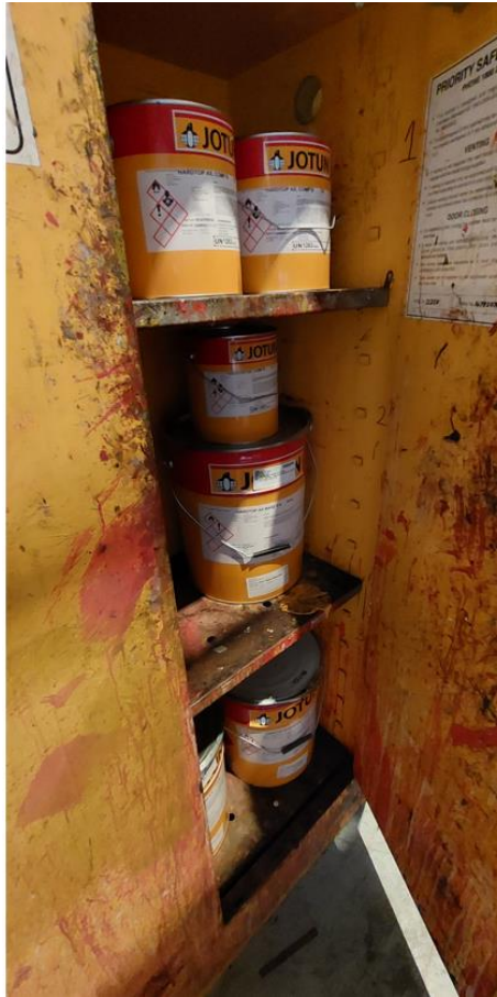
Site Photo 4 Flammables storage cupboard (Maintenance).
