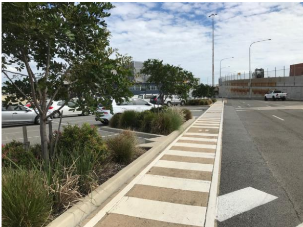
Photo 6.14.1: Maintenance car park – landscaping and sealed surface
