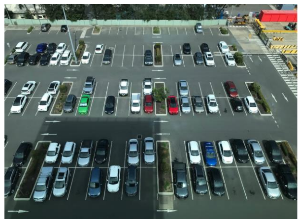
Photo 6.14.2: Main car park – landscaping and sealed surface
