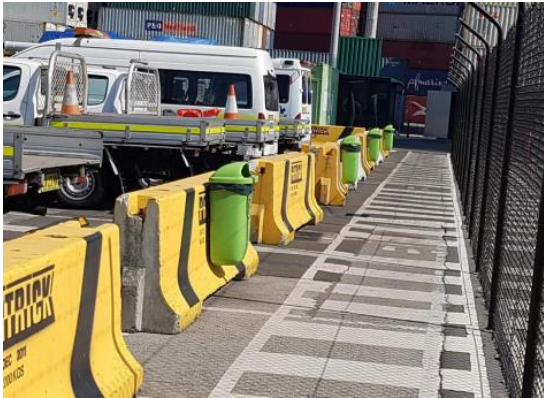
Photo 6.8.1: Enclosed rubbish bins next to Operations vehicle parking area
