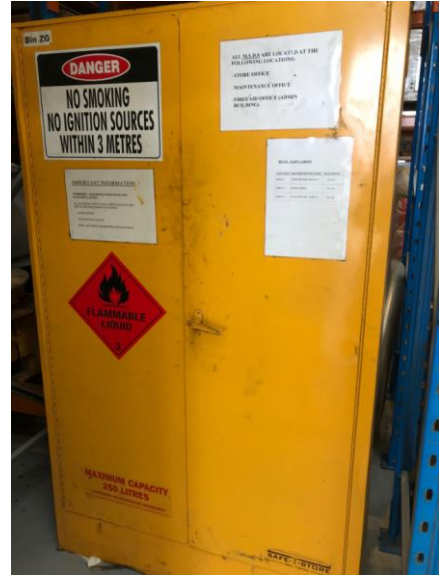
Photo 6.9.2: Flammable liquids cabinet
