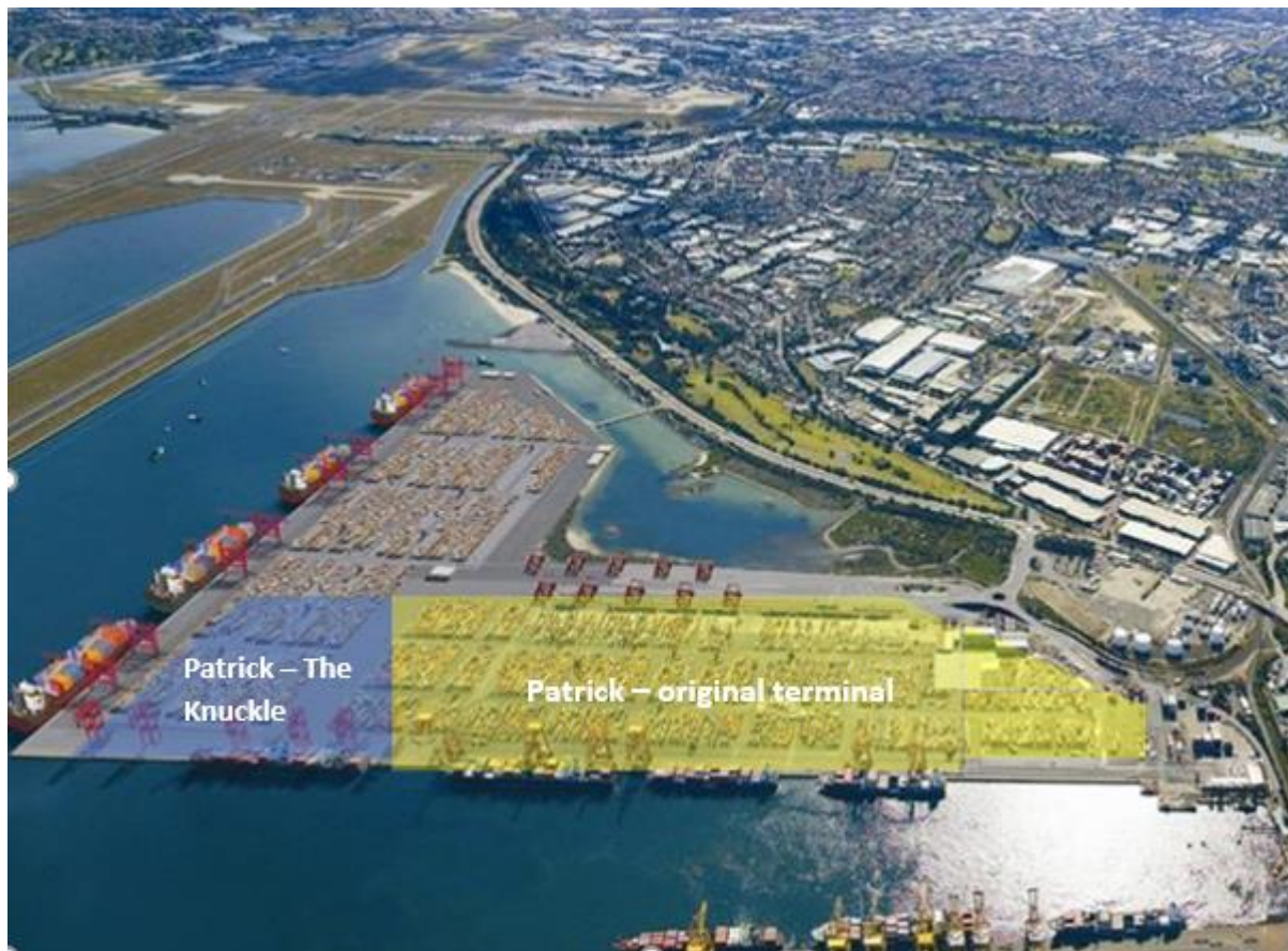
Figure 2 Patrick Stevedores site at Port Botany showing areas covered by DA 453 (original terminal) in yellow (Source: Patrick Operational Environmental Management Plan, 17 March 2023).
