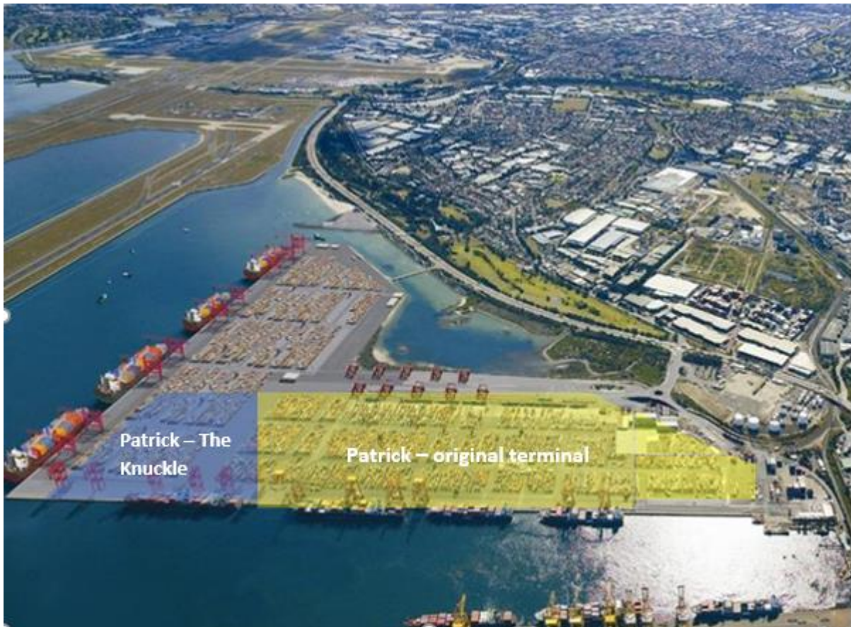
Figure 2 Patrick Stevedores site at Port Botany showing areas covered by DA 453 (original terminal) in yellow (Source: Patrick OEMP, 17 January 2025)
